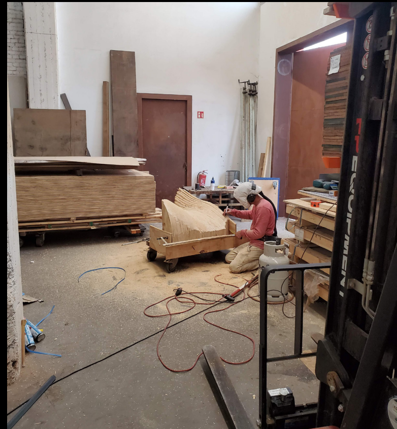
fig. 8 Valentin making the profiles for a concrete bench
